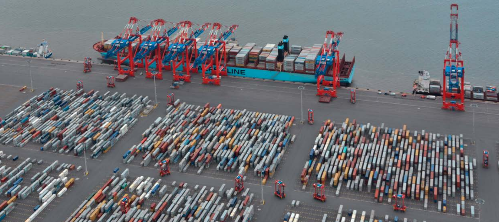
Wilhelmshaven container terminal
